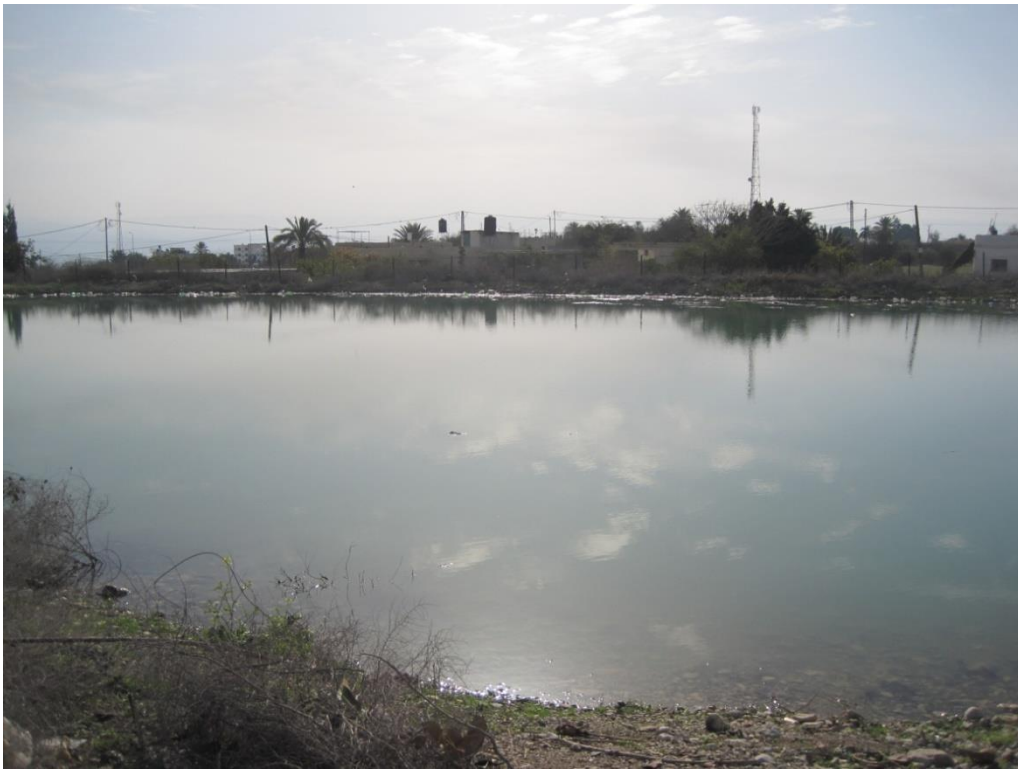
Figure 1: surface storage pond for feeding the injection borehole.
