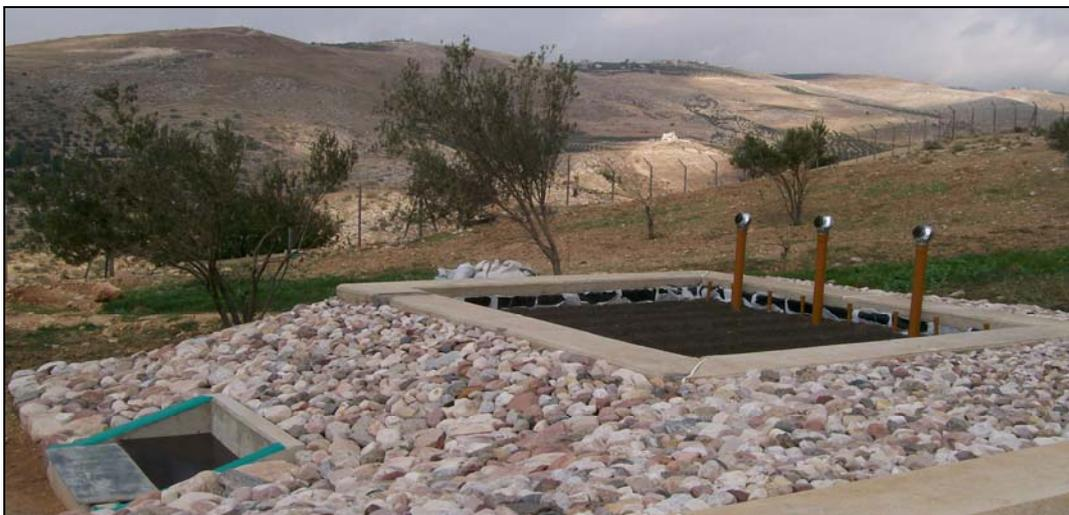
Figure 7: Photo of the recirculating treatment wetland at the Fuhais site.
