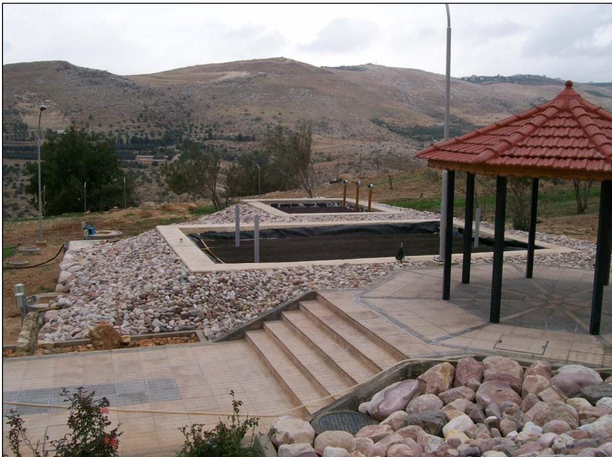
Figure 2: Photo of the treatment wetlands installed at the Fuhais site.
